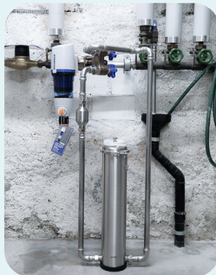
Floor Installation on a compact Y-flange.
