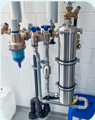
Overhead Installation using pipe clamps and a Y-flange.
