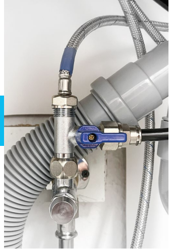
Feed water valve; with 3/8" inch GSM connector, stopcock with 3/8" water inlet connection.
